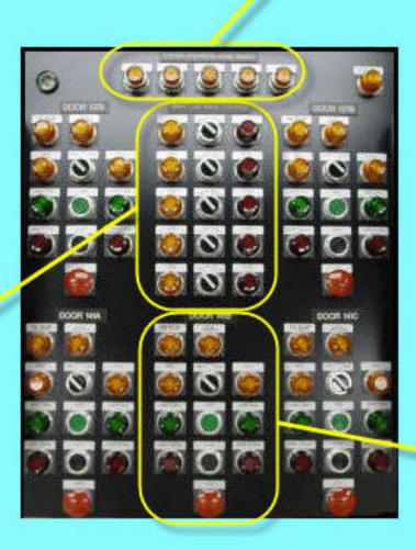
THIS FIELD OF BUTTONS, SWITCHES AND INDICATORS IS USED TO CONTROL AND ANNUNCIATE THE STATUS OF BOTH THE GRILL & DOOR AT ENTRY 141B
